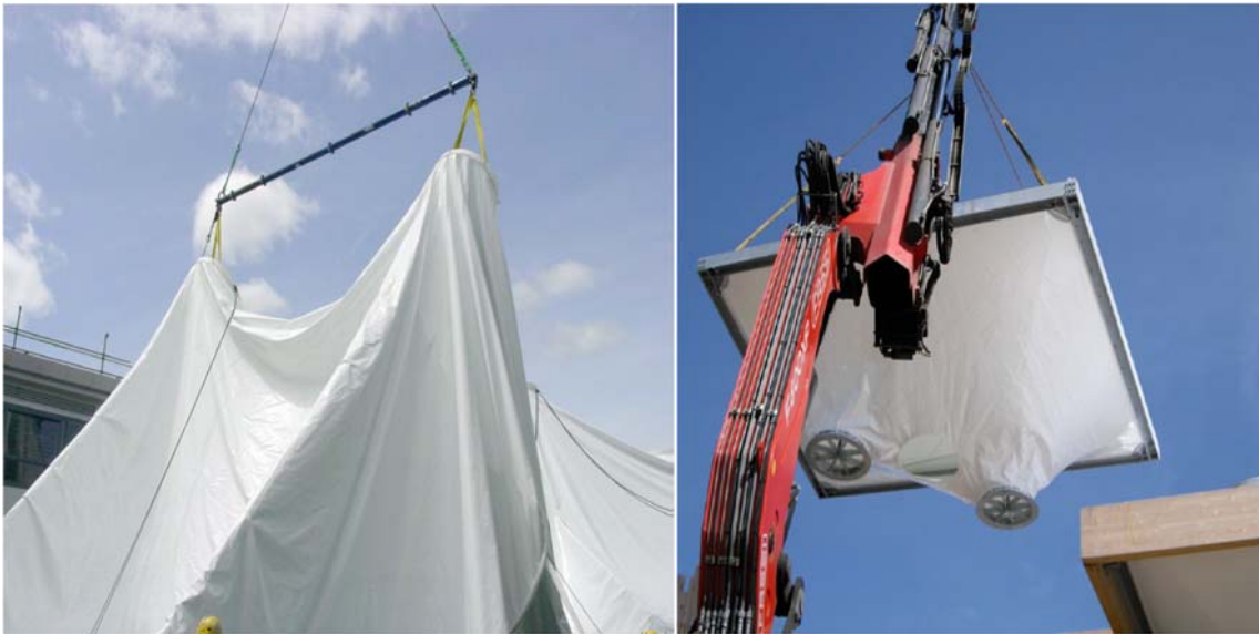
Fig.13 Erection of fabric structure
