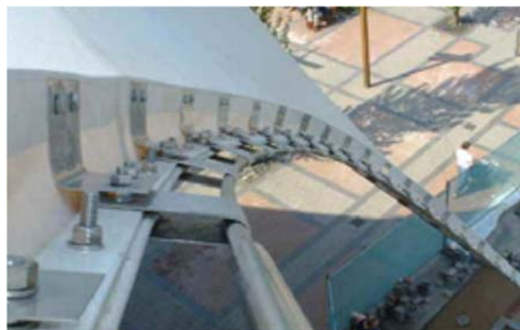
Fig.12 Boundary cable upstand plate
