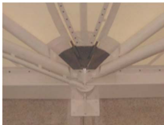
Fig.8 Fabric joined by clamping
