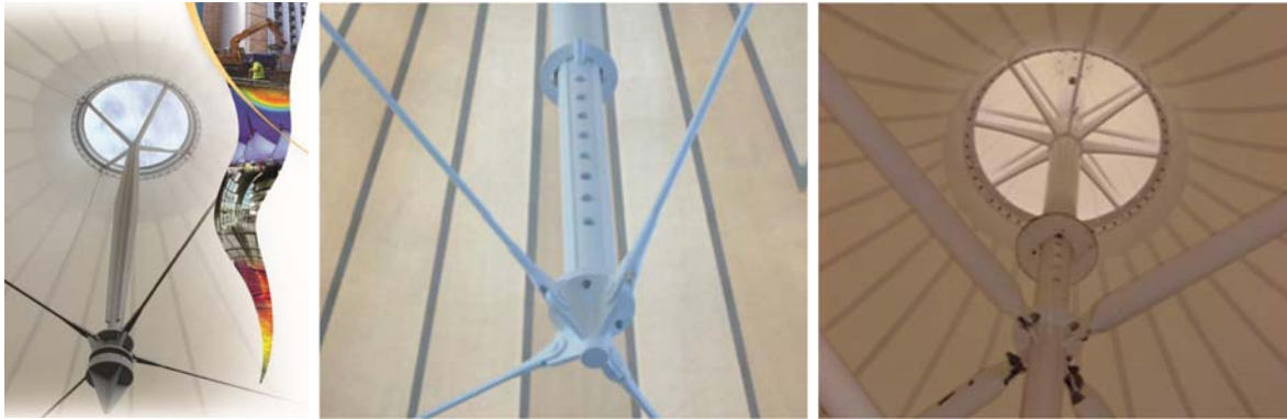
Fig.11 a) Mast, b) Flying mast & jacking system, c) Fixed mast & head ring clamping
